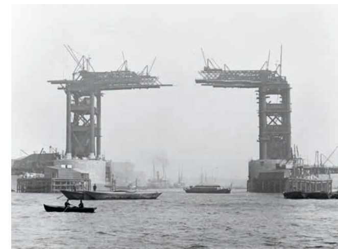
Tower Bridge under construction c.1889
