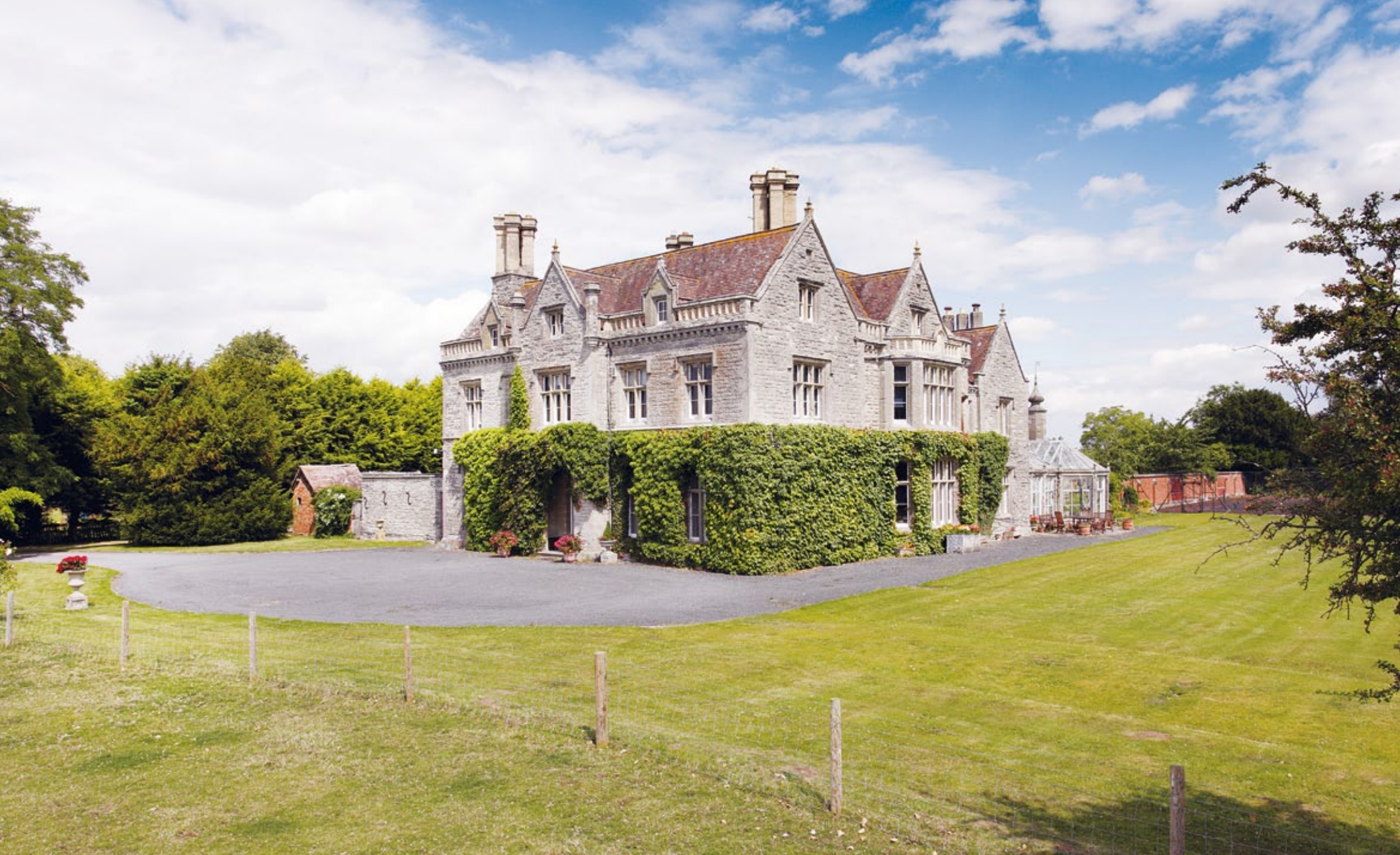
Chambers Court, Longdon, Tewkesbury, Gloucestershire
