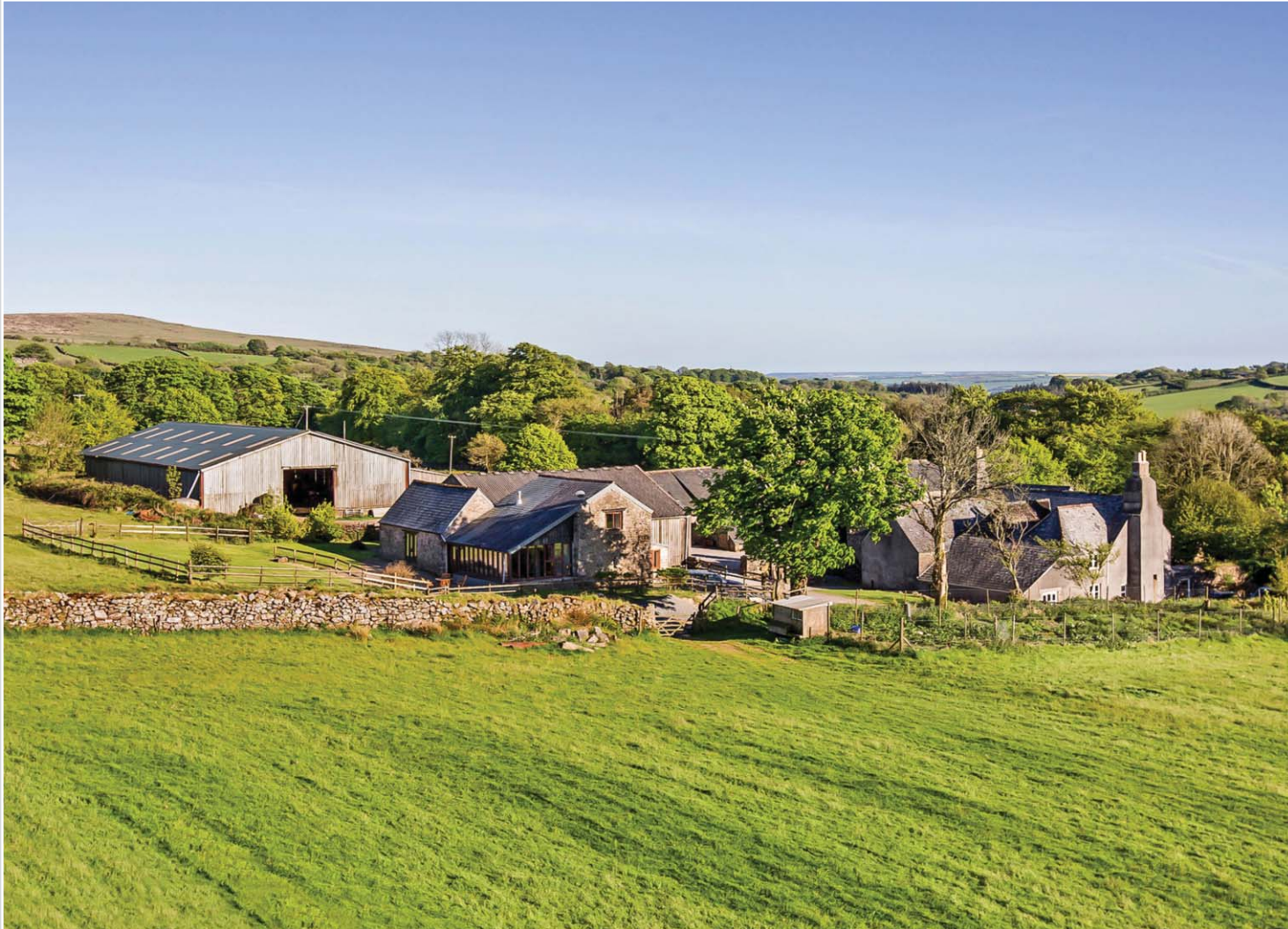
Hall Farm, Ivybridge
