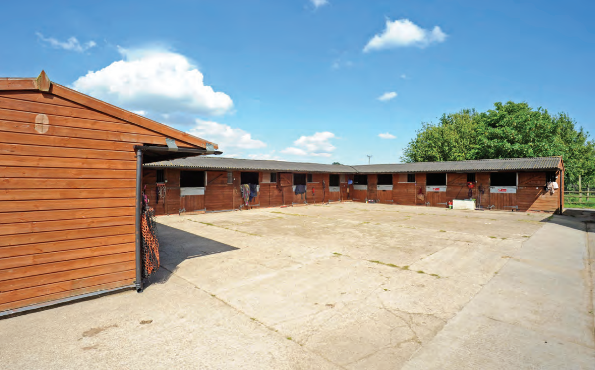
11 Lodden Stables and Courtyard
