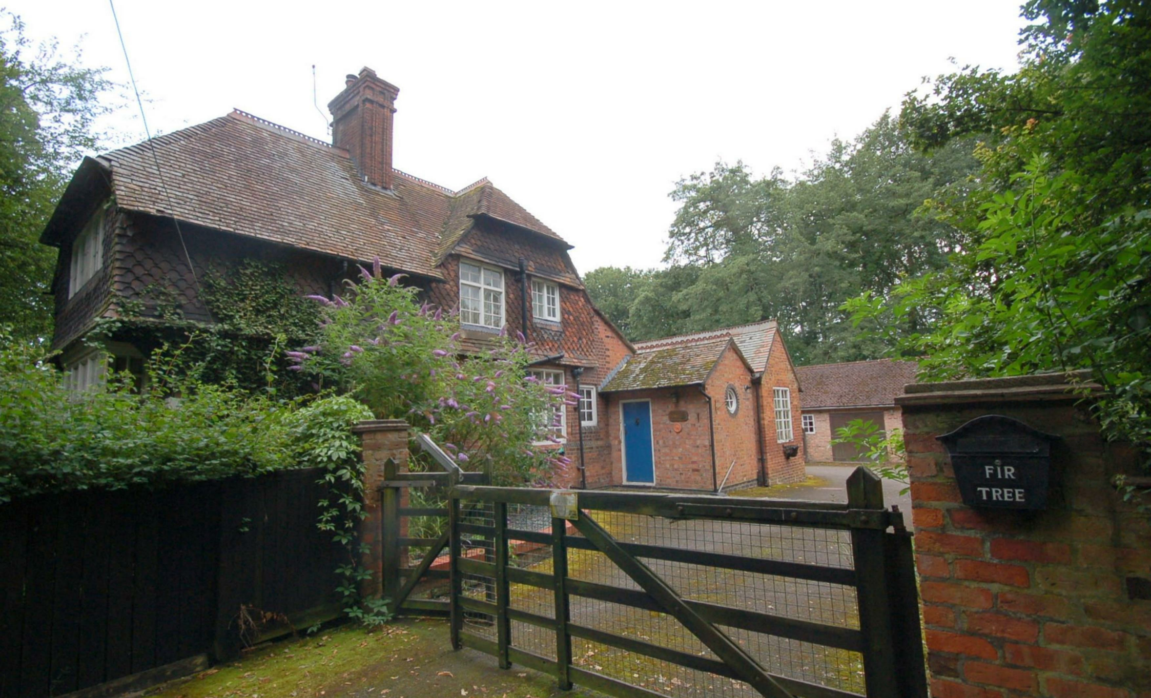
Fir Tree Cottage, Weston Road Crewe CW1 5XN Guide Price £300,000
