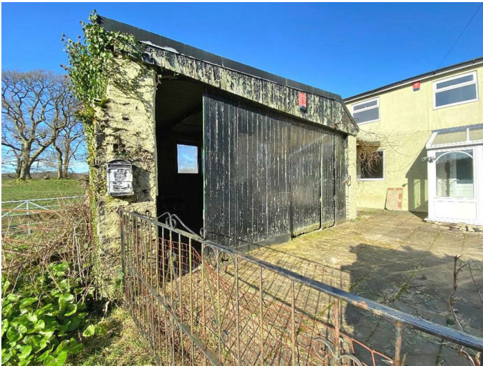
With power connected.
