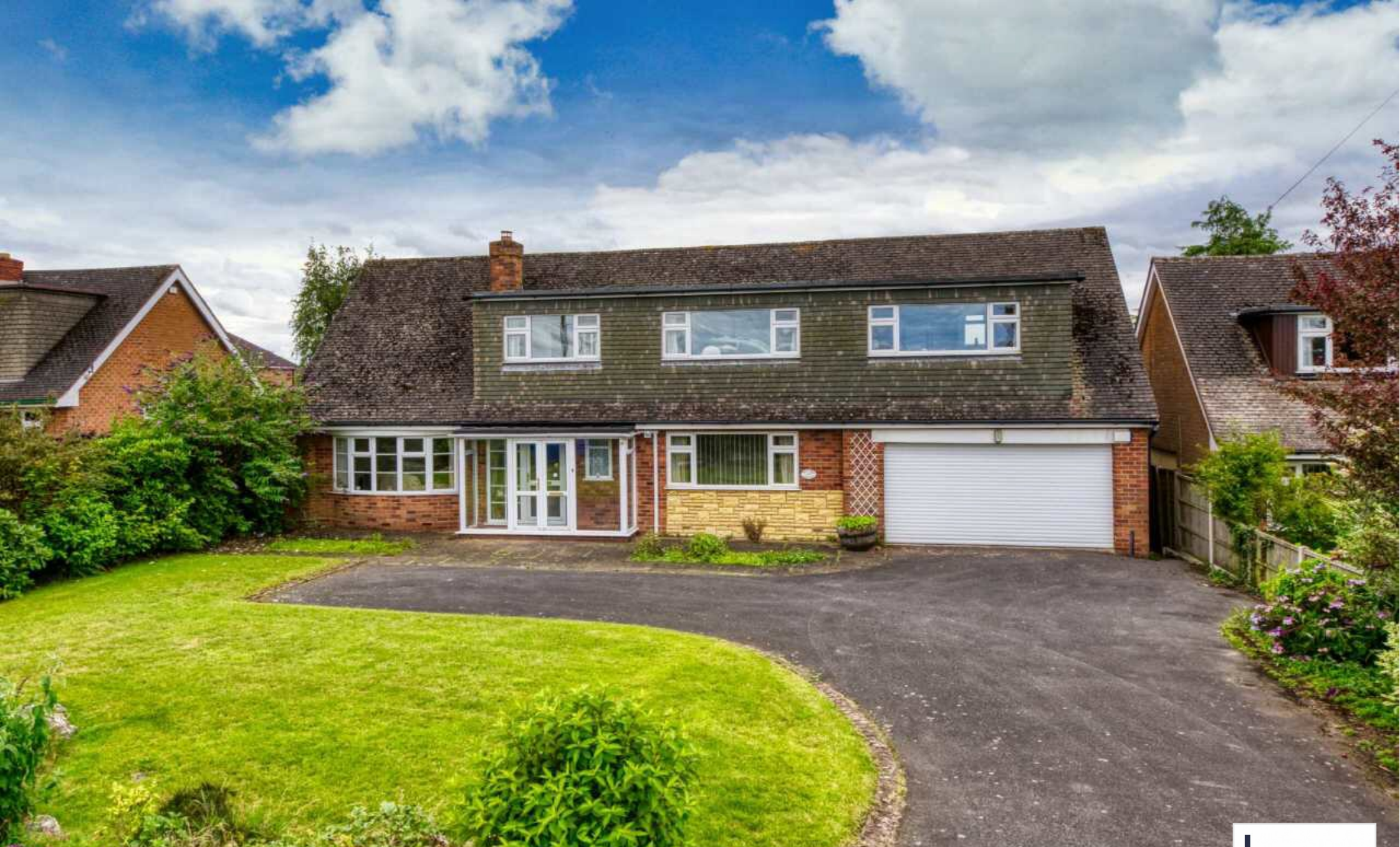
Drifters Cottage, Ivetsey Bank Road, Bishops Wood, Stafford, ST19 9AE
