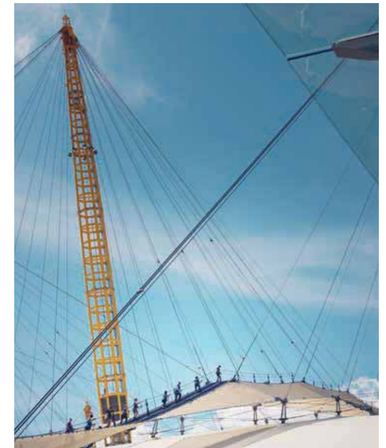
Up The O2 spans the building's canopy to give exhilarating views across London.
