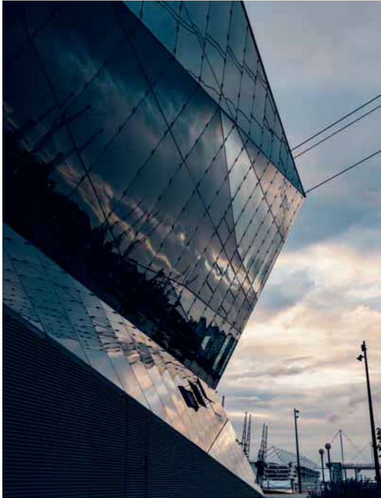
The Siemens Crystal beside the ExCel London exhibition centre encourages us to change the way we think about urban life through a glimpse into its sustainability and its future.
