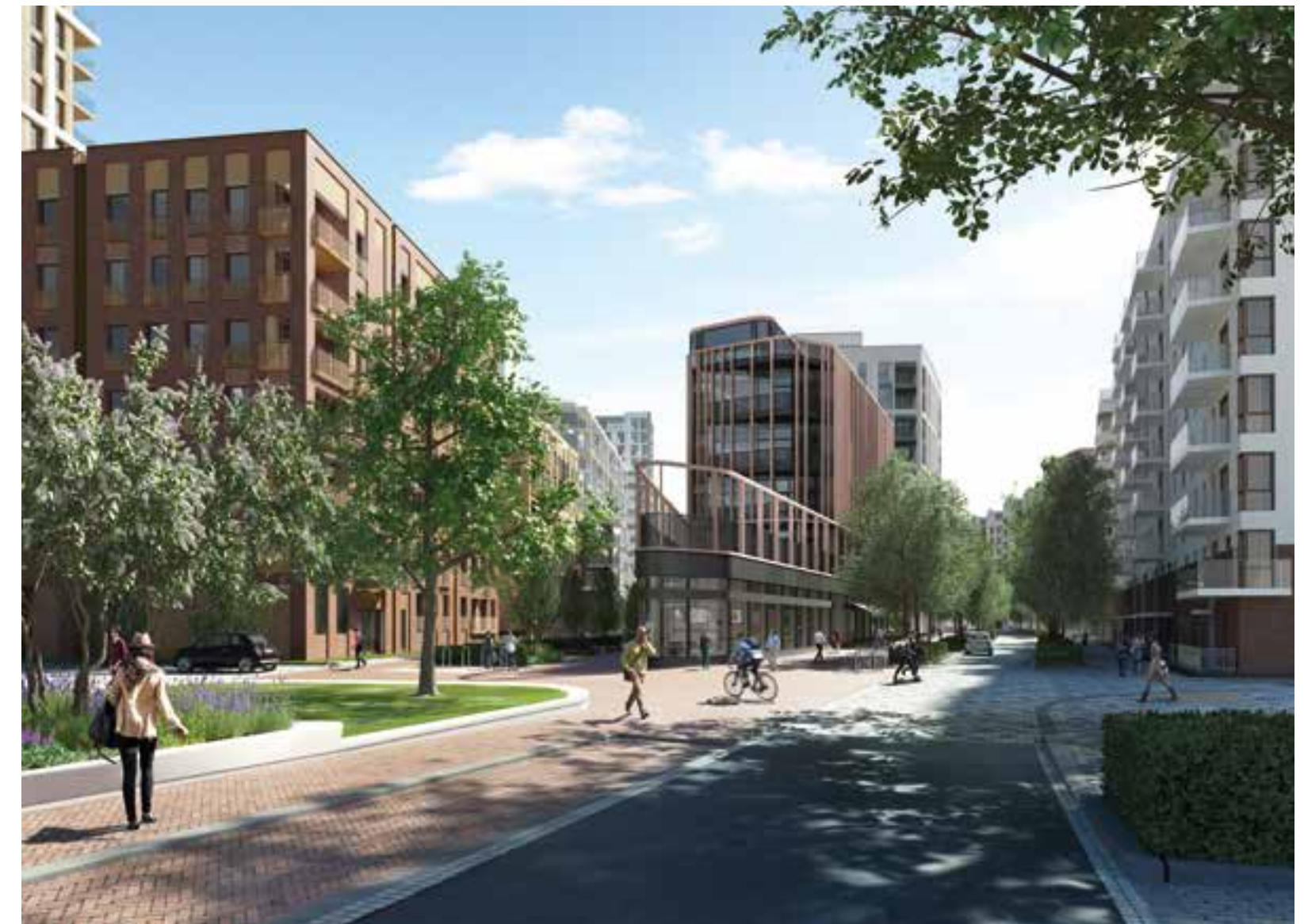
Aperture, Chandlers Avenue Greenwich Peninsula
