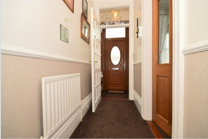
Central heating radiator.
