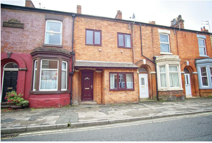
External front of house with full double glazing.
