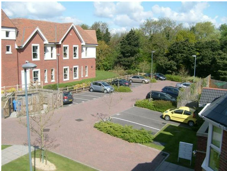
Allocated space to the rear of the property.
