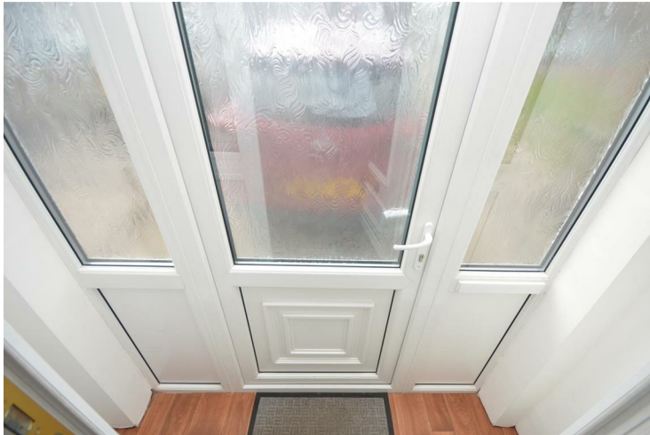
Vinyl flooring and main entrance door.
