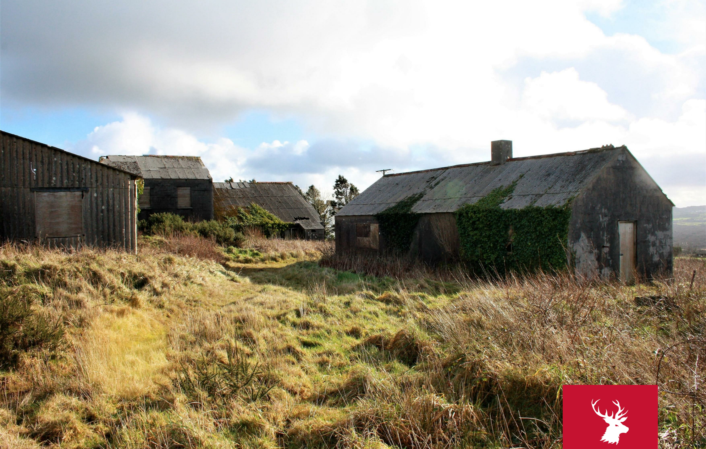
Castle an Dinas Mine Buildings
